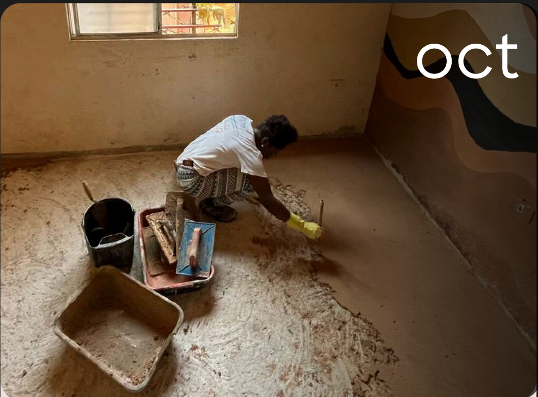
community joint-efforts: earthen floor installation
