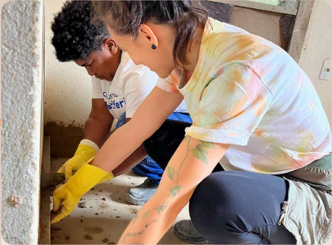
joint efforts: earthen baseboard installation
